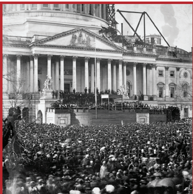
Lincoln swearing-in at the partly finished Capitol building.
